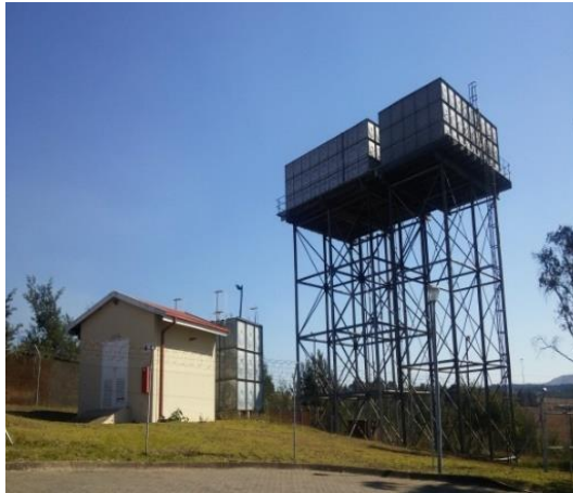
Figure 3-1: Two elevated potable water tanks, a firewater tank and a fire pump station
