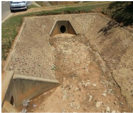
Figure 3-7: Grouted stone pitching with silt deposition
