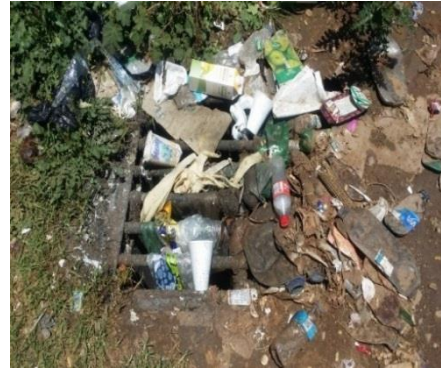
Figure 3-6: Blocked grid inlet
