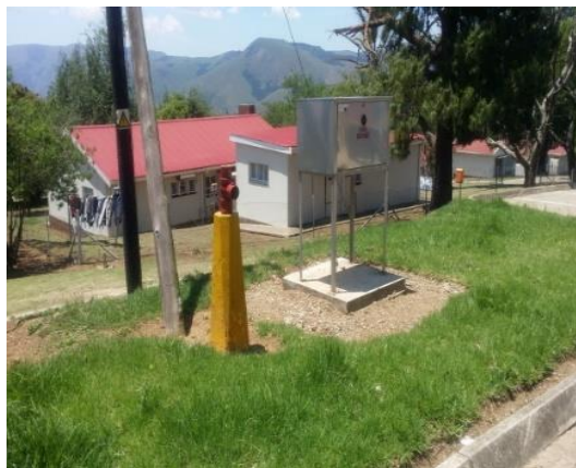
Figure 3-3: Firewater hydrant and hose reel
