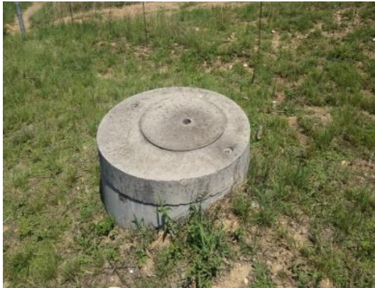
Figure 3-4: Non-overflowing sewer manhole
