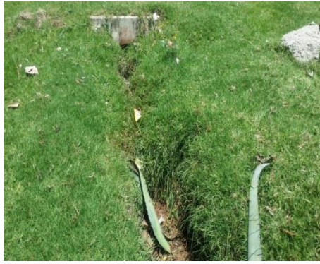
Figure 3-5: Earth channel overgrown with grass
